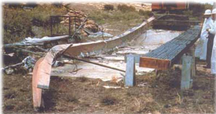
Above: Equivalent strength steel beam and glulam beam following fire test under full load. Steel beam collapsed after only 30 minutes exposure, while glulam member remained straight and true, charring only 3/4" on exposed surfaces.
