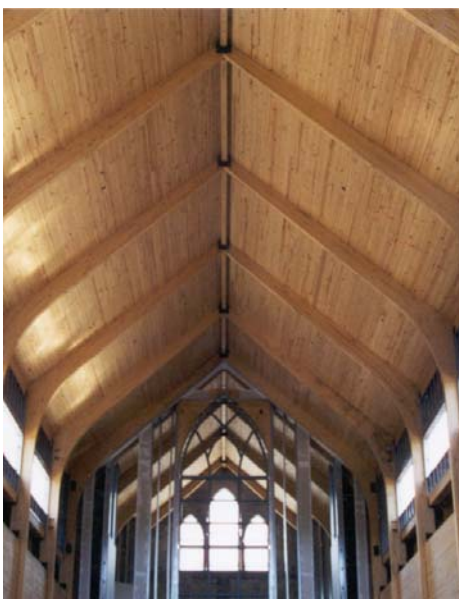
Church, Palm Beach Gardens, Fla., Unit Structures
