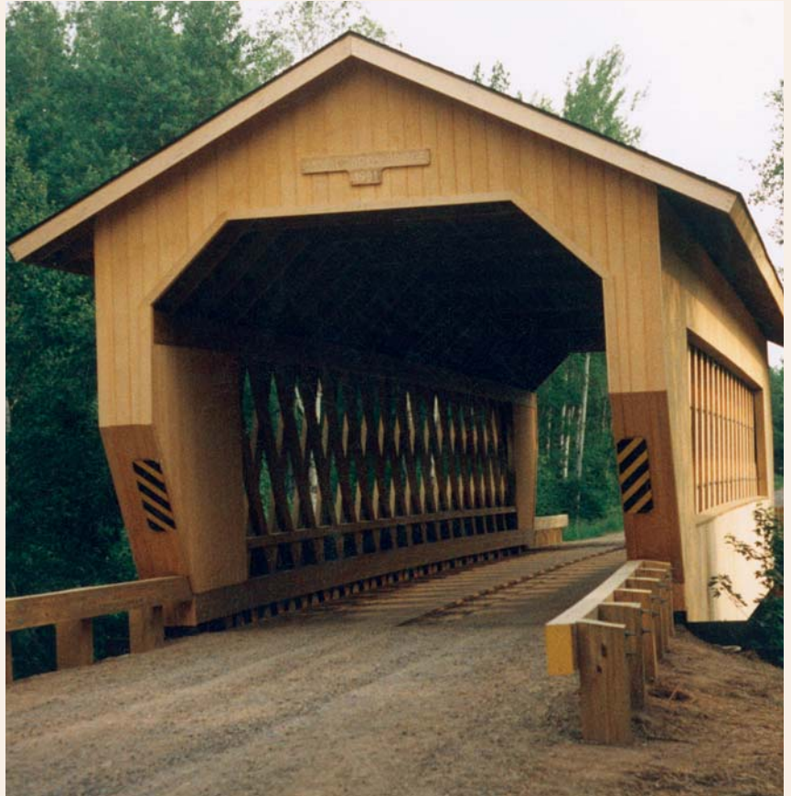
New covered bridge with laminated trusses. ENGINEER: USDA Forest Service.
