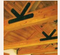
Truss connection.
