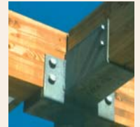
Beam intersection connection.
