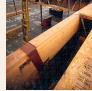
Cantilever connection.
