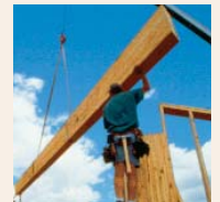
Installing a residential ridge beam.
